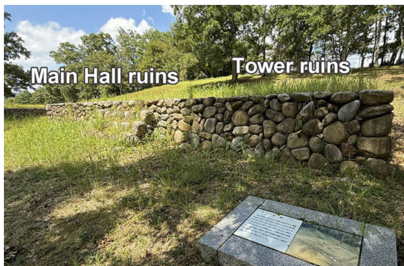
Foundation of the pagoda at Natsumi Temple (Shōfuku-ji) — the Lecture Hall and Pagoda were completed in 725
