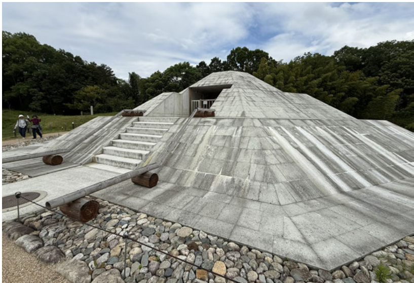
Kengoshizuka Tumulus, where Empress Saimei and Princess Hashihito are said to have performed music together (Takaichi District, Nara Prefecture)
